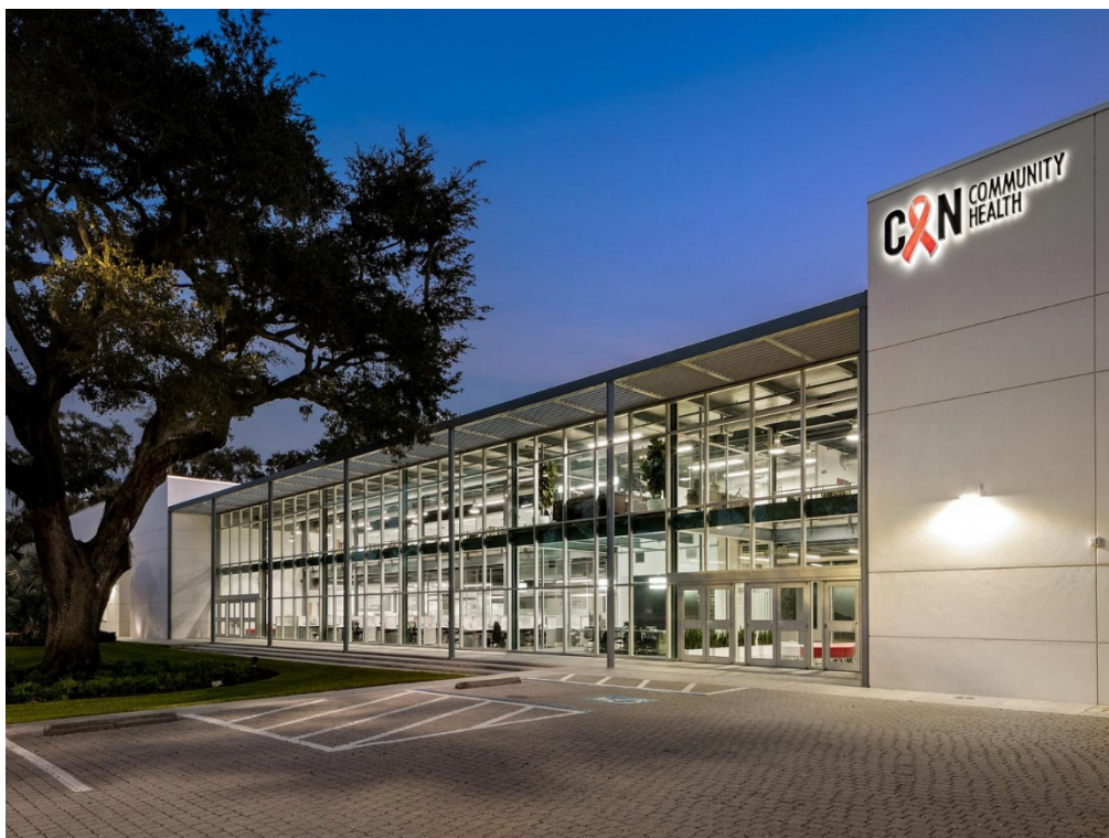
Sarasota, Florida Headquarters Building
