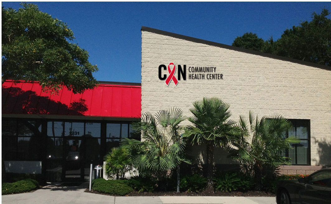
Sarasota, Florida Clinic Facility
